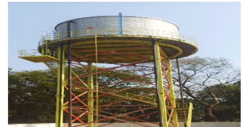
Water Tank, Uttar Pradesh
